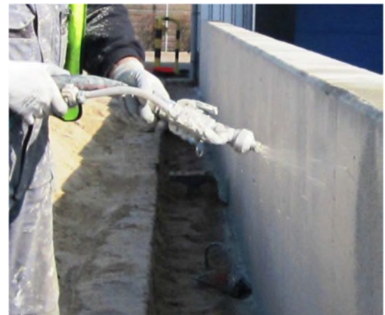
Image 2: Spray application of MasterSeal 6100
