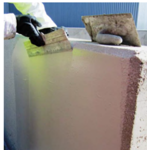
Image 3: Finish of MasterSeal 6100 FX application
